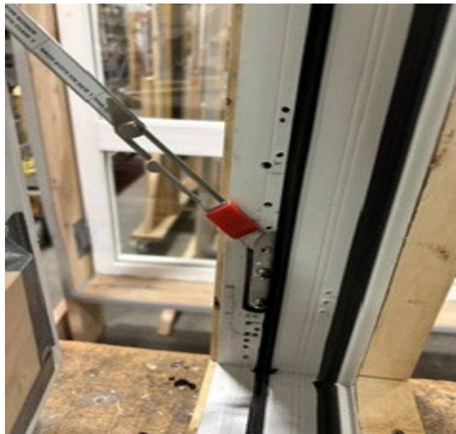
Photo No. 2 WOCD engaged secured to Jamb
